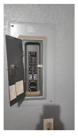
9.2.2 Main Panel Service & Grounding, Main Overcurrent Device
